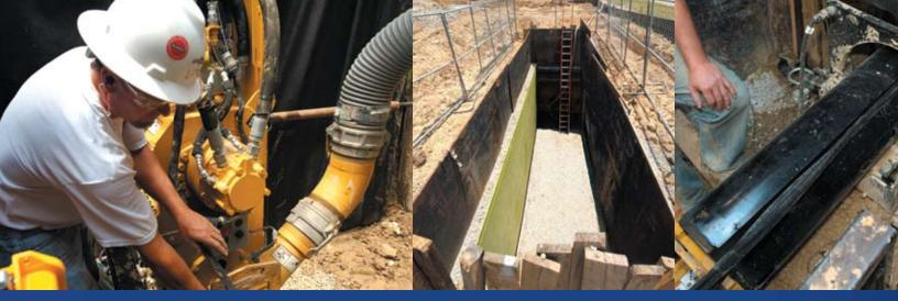
**RESTORATION COSTS** — The AXIS guided boring system is designed to help minimize restoration costs compared to other methods. It requires surface excavation for two pits that can serve as the manhole locations, saving additional excavation time and resources. When compared with open cut, the AXIS system significantly decreases surface restoration costs.
